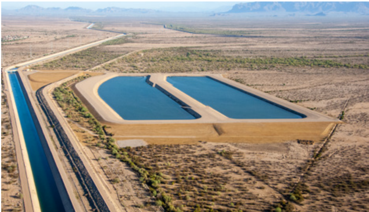
Superstition Mountains Recharge Project
