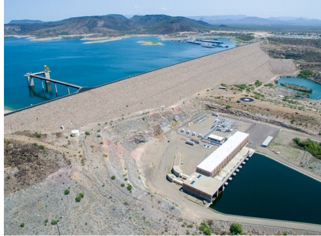
Hydroelectricity at New Waddell Dam
