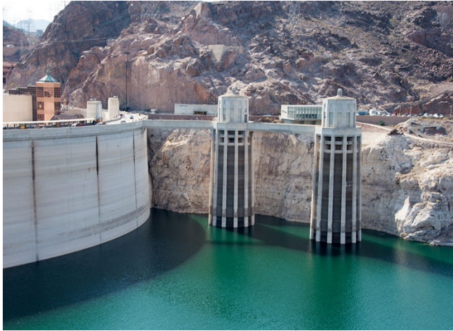
Hydroelectricity at Hoover Dam
