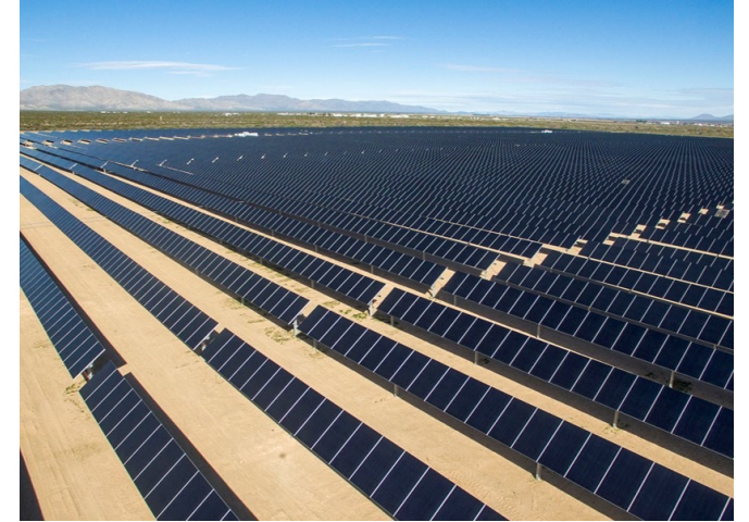
Solar Power at Origis Energy Solar 1 Project
