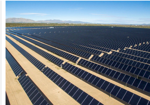
Solar Power at Origis Energy Solar 1 Project
