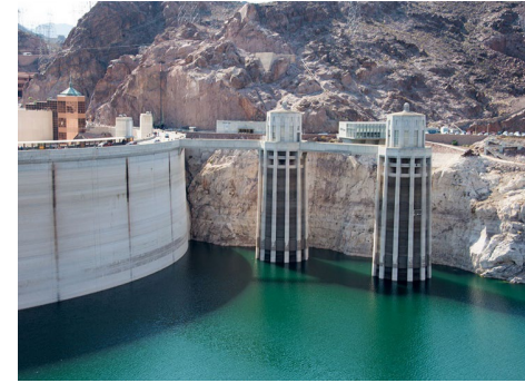
Hydroelectricity at Hoover Dam
