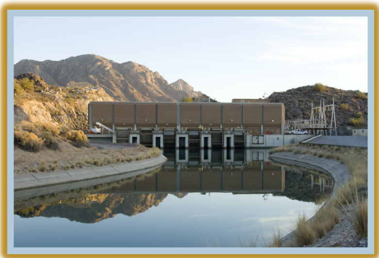
Picacho Pumping Plant
