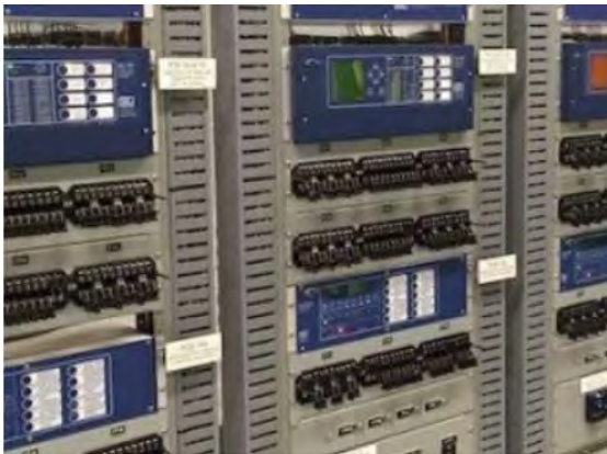
Electromechanical Relay Replacements Phase 2
