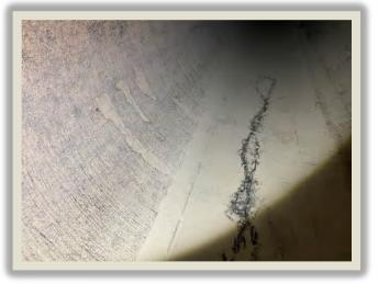
concrete exposed can lead to spalling of the concrete and potential damage to the impellers.
