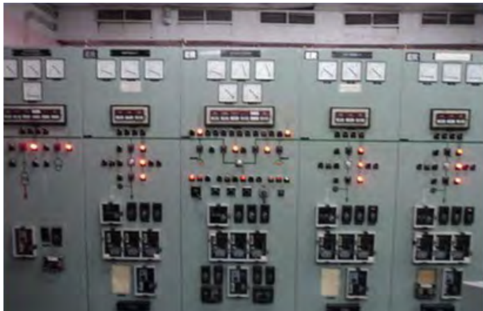
Electromechanical Relay Replacements Phase 2
