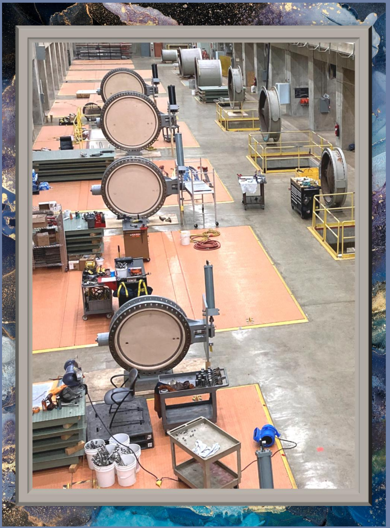
Inside Bouse Hills - Discharge Valve Replacement
