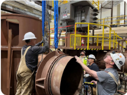
The Heavy Overhaul Team works to disassemble Unit 5 at Twin Peaks Pumping Plant as part of the planned overhaul of this unit.
