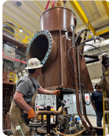
The Heavy Overhaul Team works to disassemble Unit 5 at Twin Peaks Pumping Plant as part of the planned overhaul of this unit.
