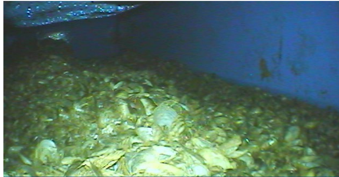
A videoscope photo of quagga mussel settlement in the cooling water header boxes at MWP. This level of infestation clogs the cooling tubes and prevents the motor from being properly cooled, eventually causing the motor to trip due to overheating.
