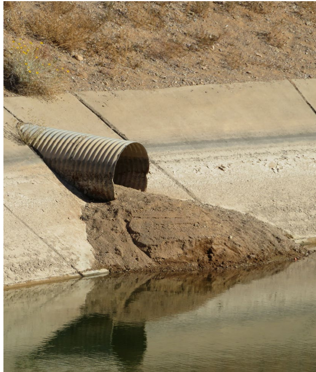
SEDIMENT FROM RUNOFF ENTERS THE CANAL THROUGH DRAINAGE STRUCTURES
