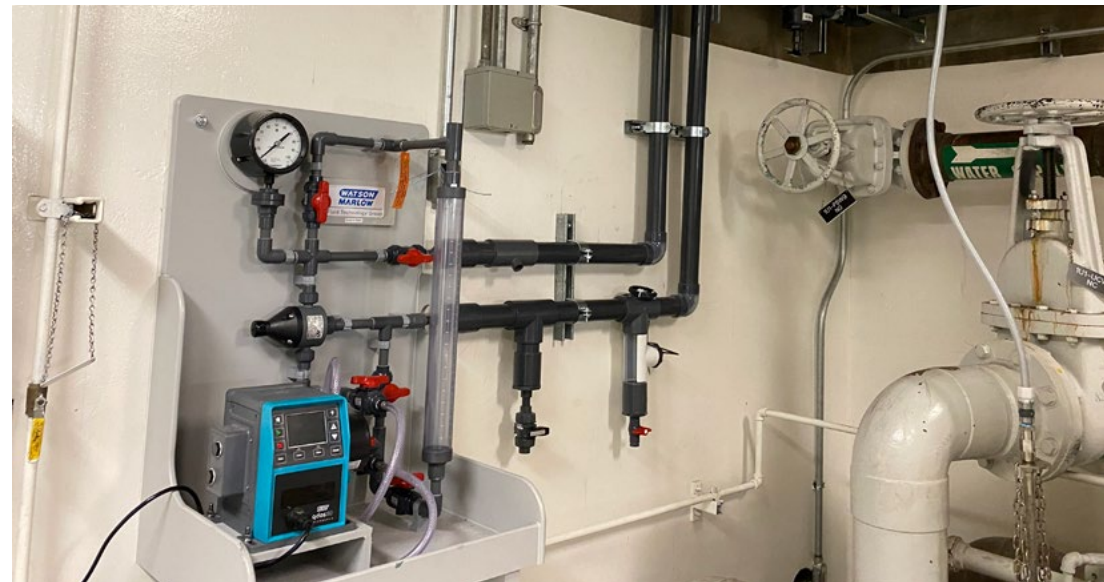
A chemical injection system has been installed on each of the six unit cooling water systems at MWP to help prevent biofouling and subsequent overheating of the motors.
