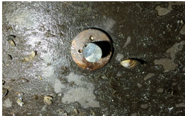
Example of a flowmeter that can get fouled by sediment deposition and quagga attachment
