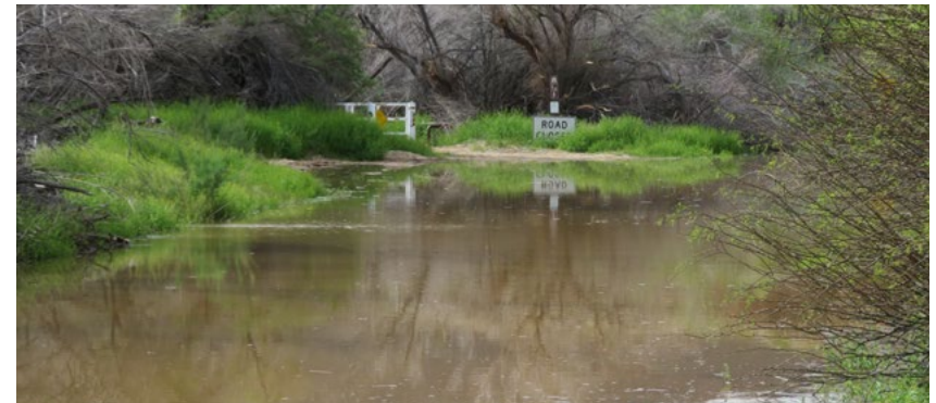
Planet Ranch Road is flooded just upstream of Lake Havasu when Alamo Dam is discharging.
