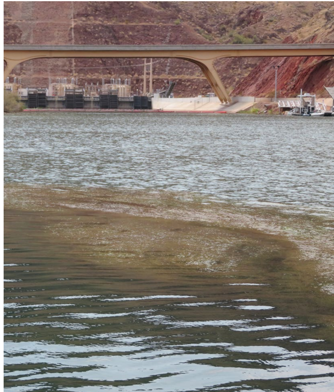
FLOATING WEED MATS APPROACH MWP DURING SUMMER MONTHS
