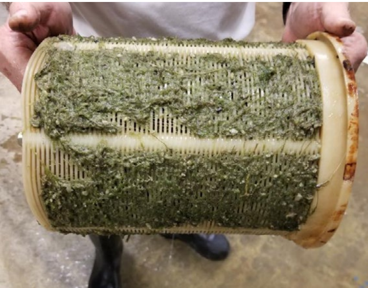
Algae fouling on a filter at LHQ in August 2020.
