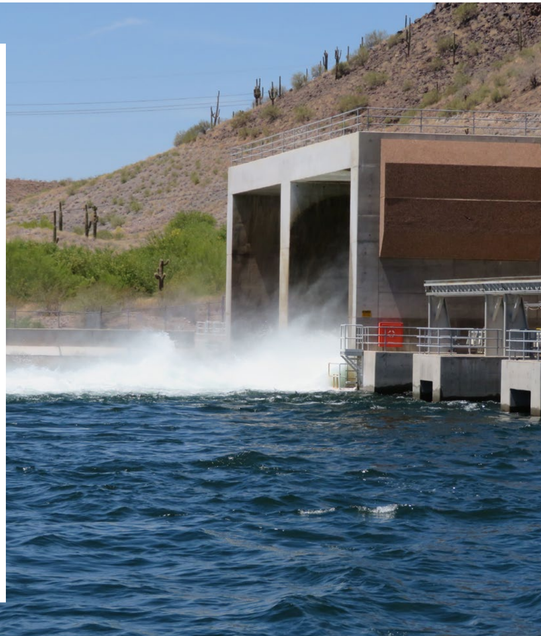
WAD BYPASS STRUCTURE Photo by Scott Bryan
