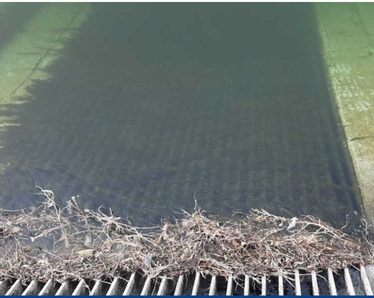
Filamentous algae and debris builds up on turnout grates and could potentially restrict flow.
