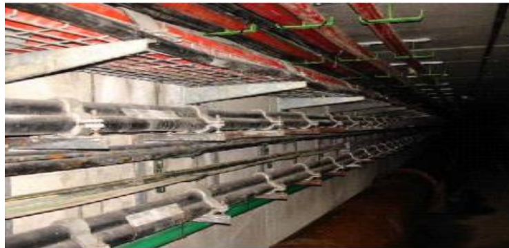
Figure 1: Power cables and communication cables in a Madrid Tunnel
