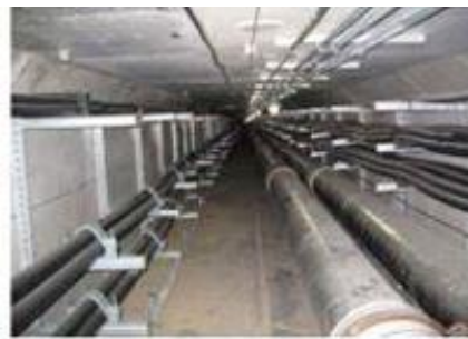
Figure 2: Typical Multi-purpose Tunnel in Stockholm
