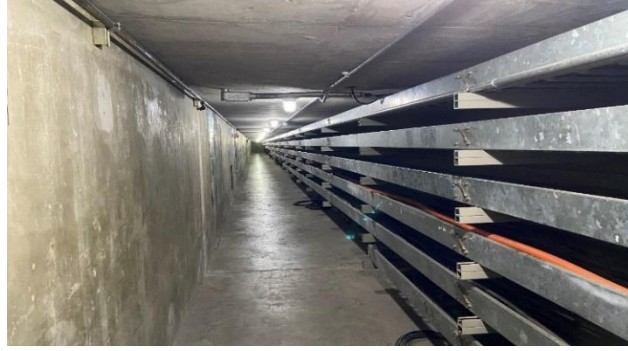
Figure 6. Cable tunnel for multiple utilities
