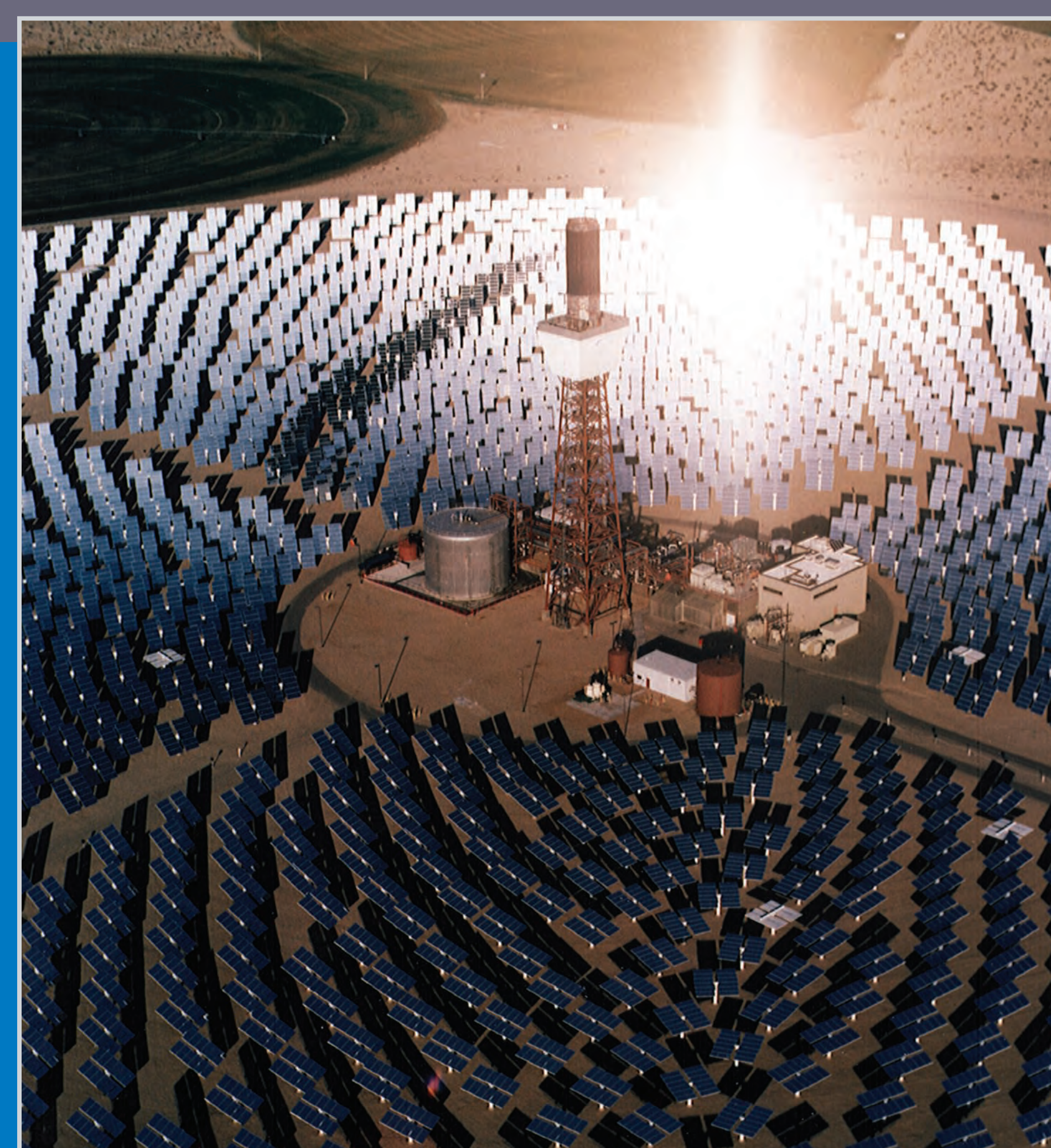
This 10-MW power tower facility known as Solar Two near Barstow, California, demonstrated molten salt storage.
