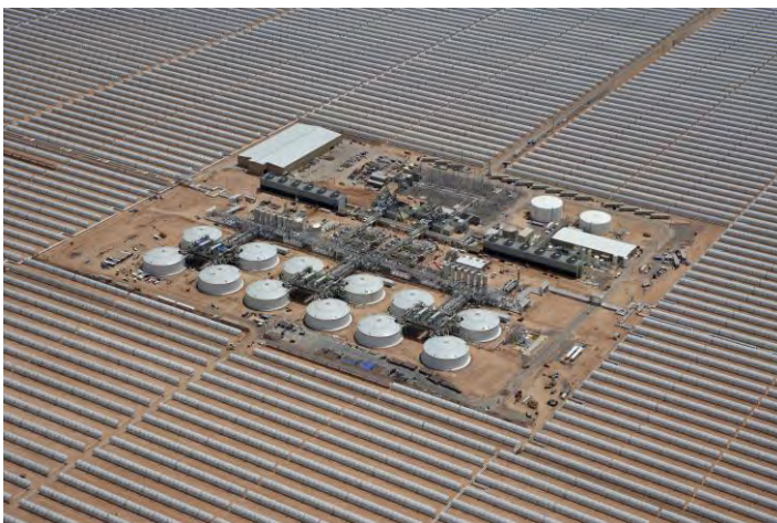
Solana's power block
