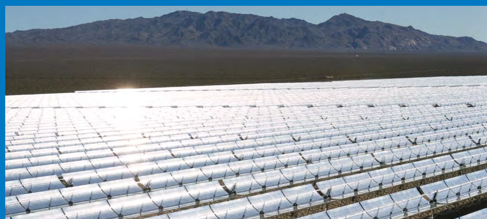
Nevada Solar One is the 3rd largest parabolic solar power plant in the world.
