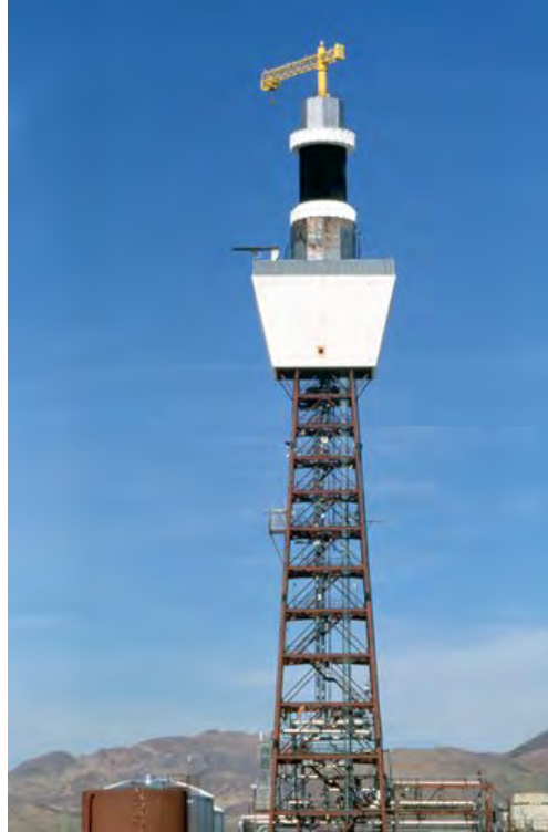
Figure 12. The Solar Two system in California included a thermal energy storage system
