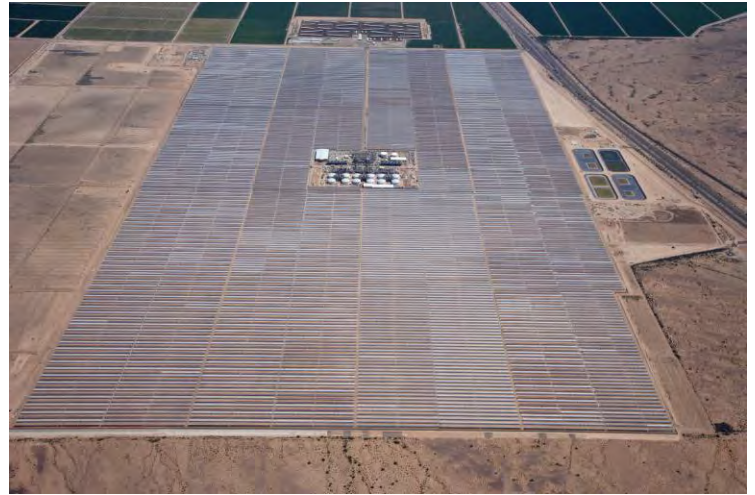
Aerial view of the solar field Photo taken July 2013
