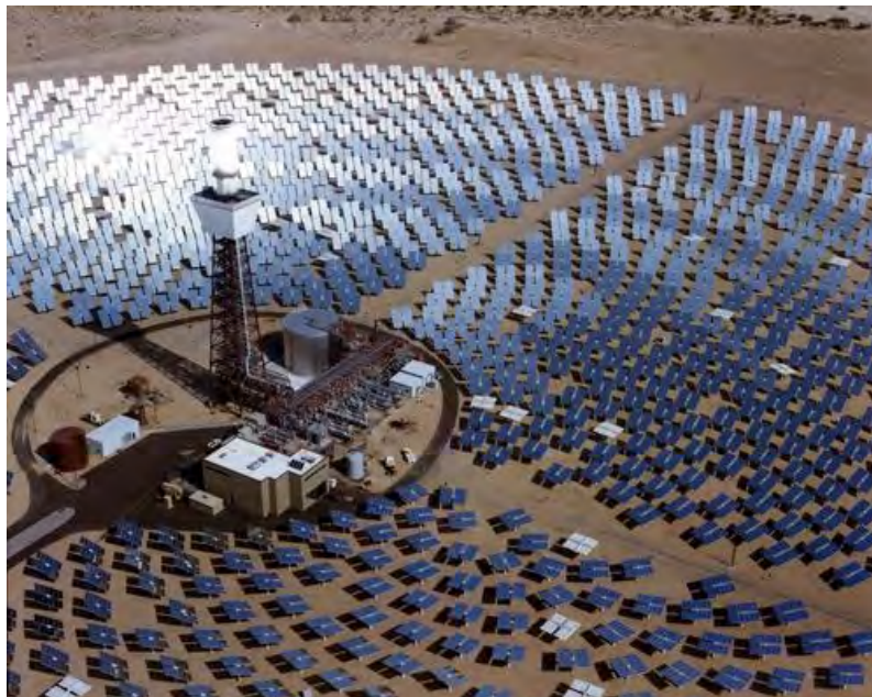
Figure 7. The Solar One facility in California employed CSP tower technology
