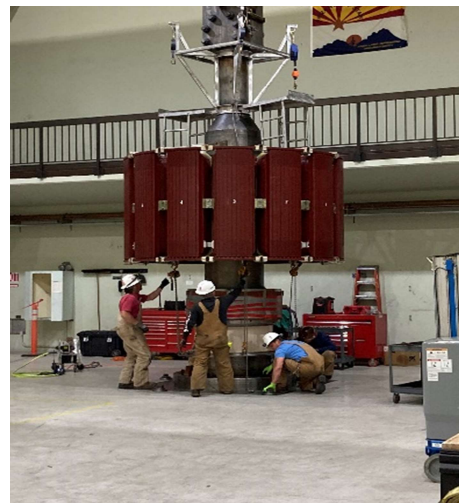
MWP Unit 5 Pole Replacement
