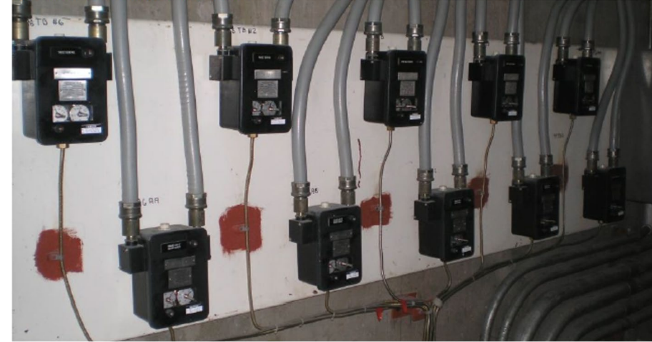
Motor Thermal Relays
