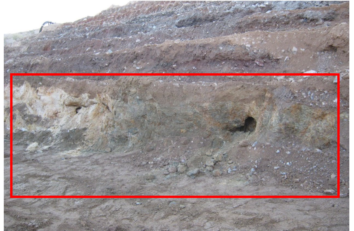
POOR FOUNDATIONAL MATERIALS
